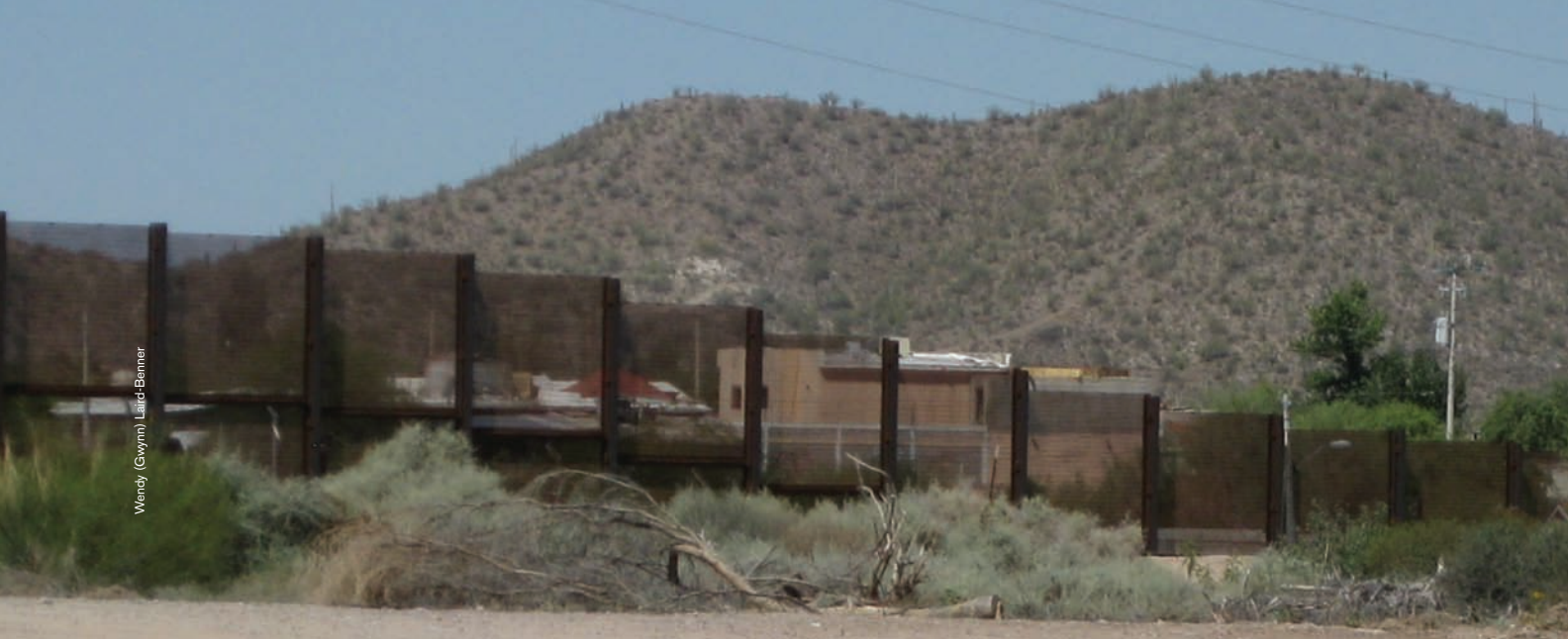
Pedestrian barrier along the US-Mexico border at Lukeville, Arizona, adjacent to Organ Pipe Cactus National Monument.
